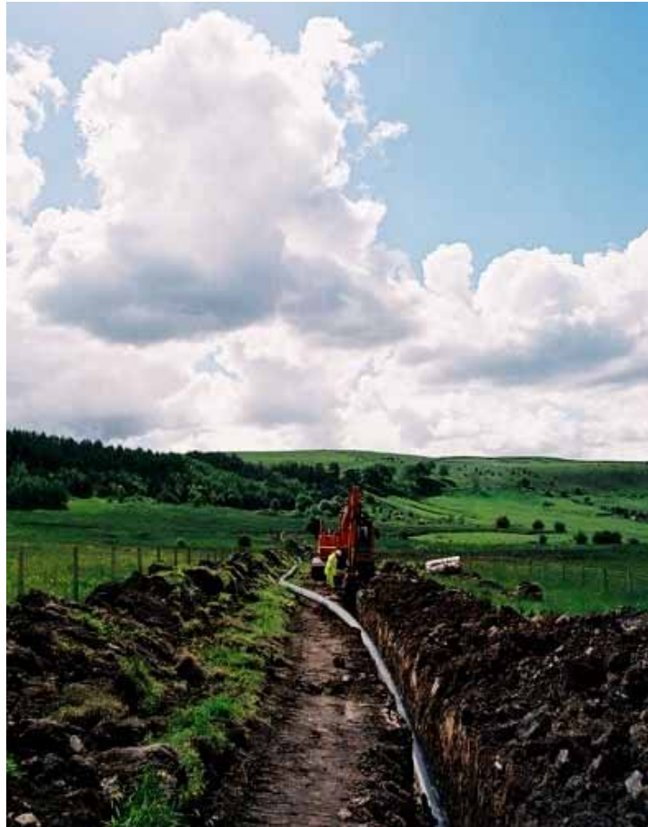
Plate 3: Topsoil stripping within the pipeline easement
