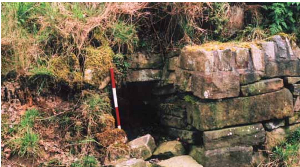
Plate 4: Culvert 161 on Ogden Lane, facing south
