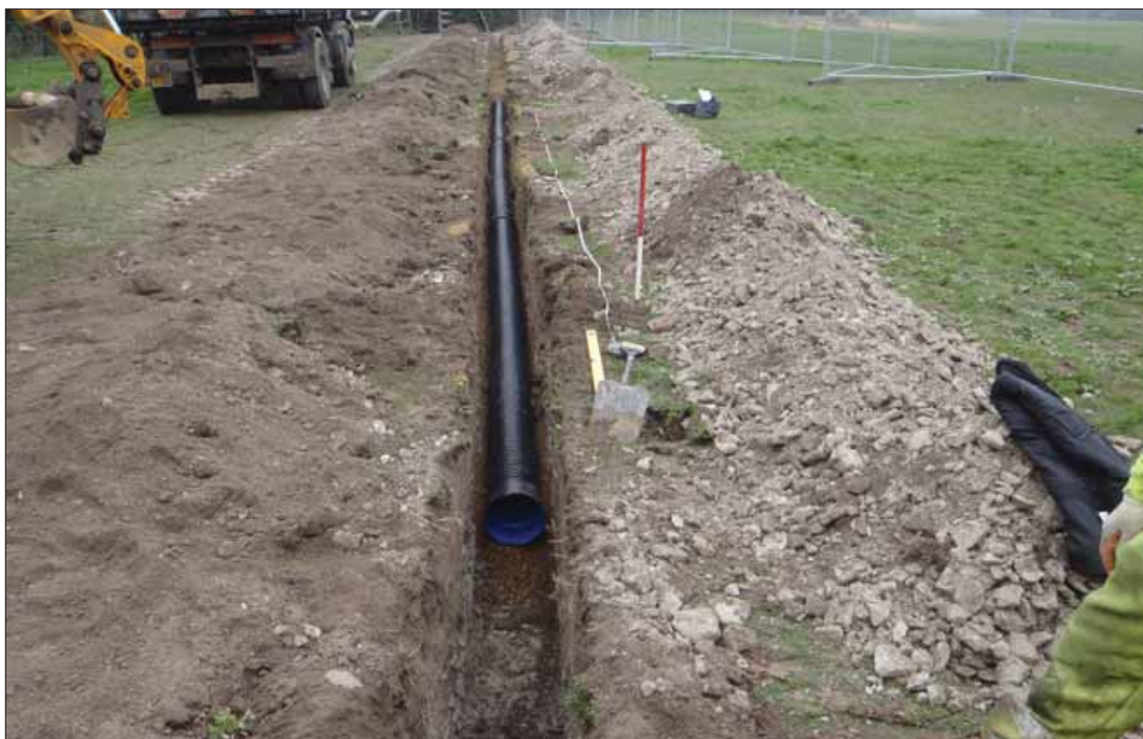
Plate 3: Part of excavated pipe trench
